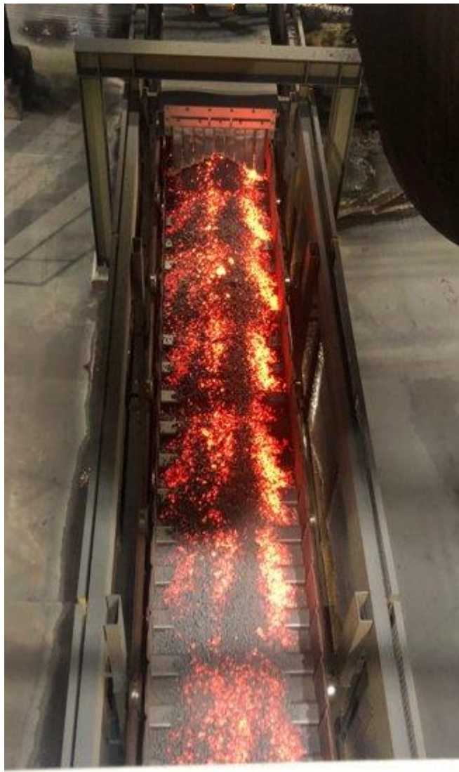
Steel Pan Conveyor transporting hot pellets
