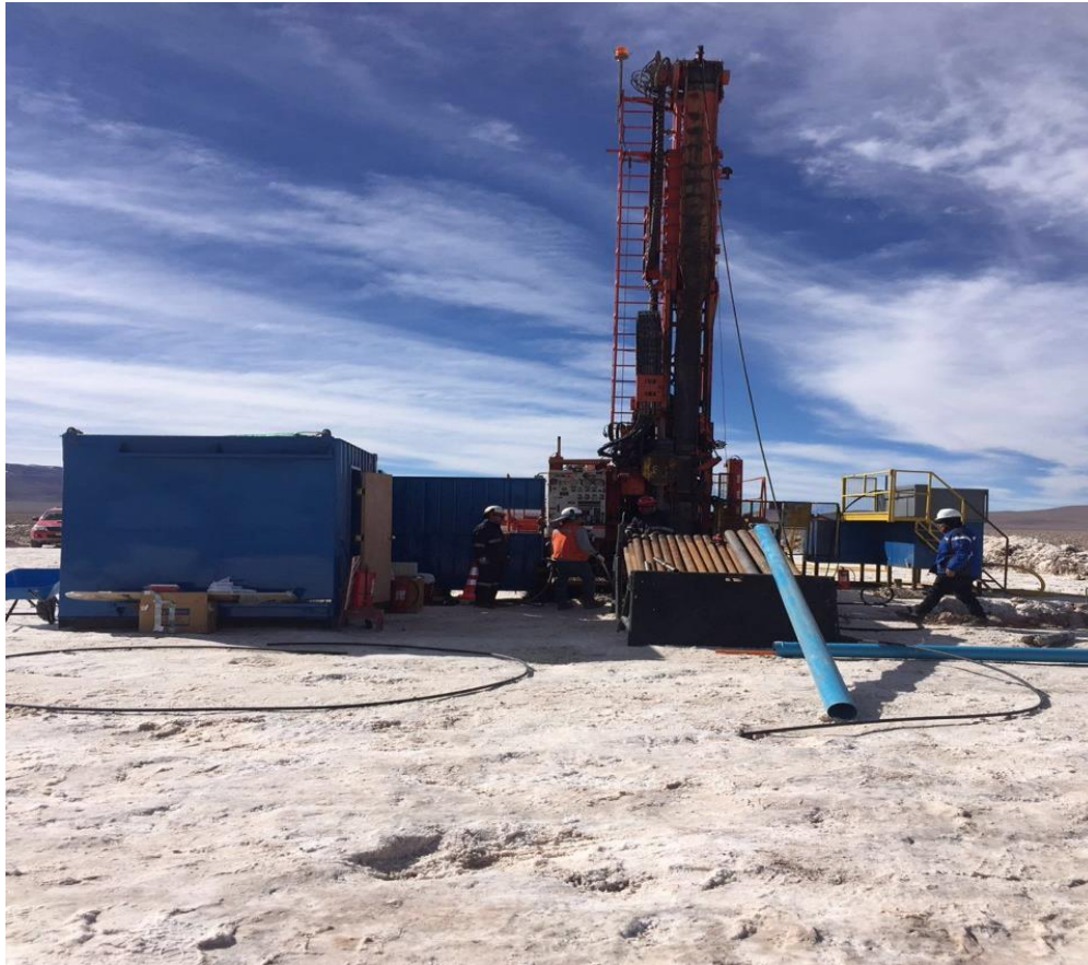
Figure 3 - Drilling of the S19 borehole to 362 m in the 2018-19 drilling program
