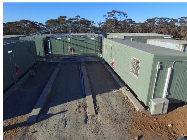
Cassini site set-up (anti-clockwise) – aerial views of site, box-cut ramp, and final footings for veranda area at office complex
