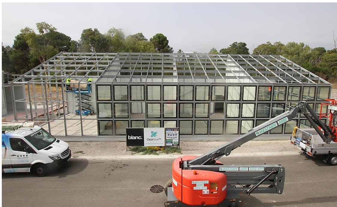
ClearVue's PV glazing being installed onto ClearVue's solar greenhouse at Murdoch University, Western Australia.
