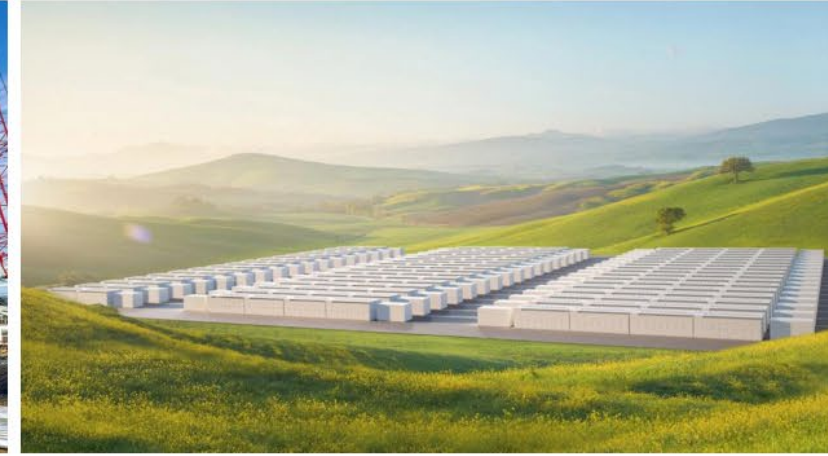
Moss Landing Energy Storage California
