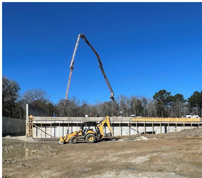
Figure 1. Atlantic Waste Services new waste transfer station
