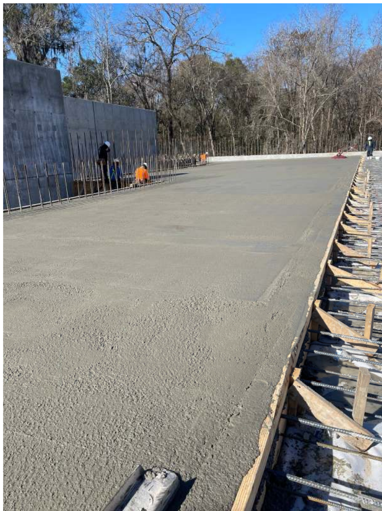
Figure 3. EdenCrete® enhanced concrete slab being installed
