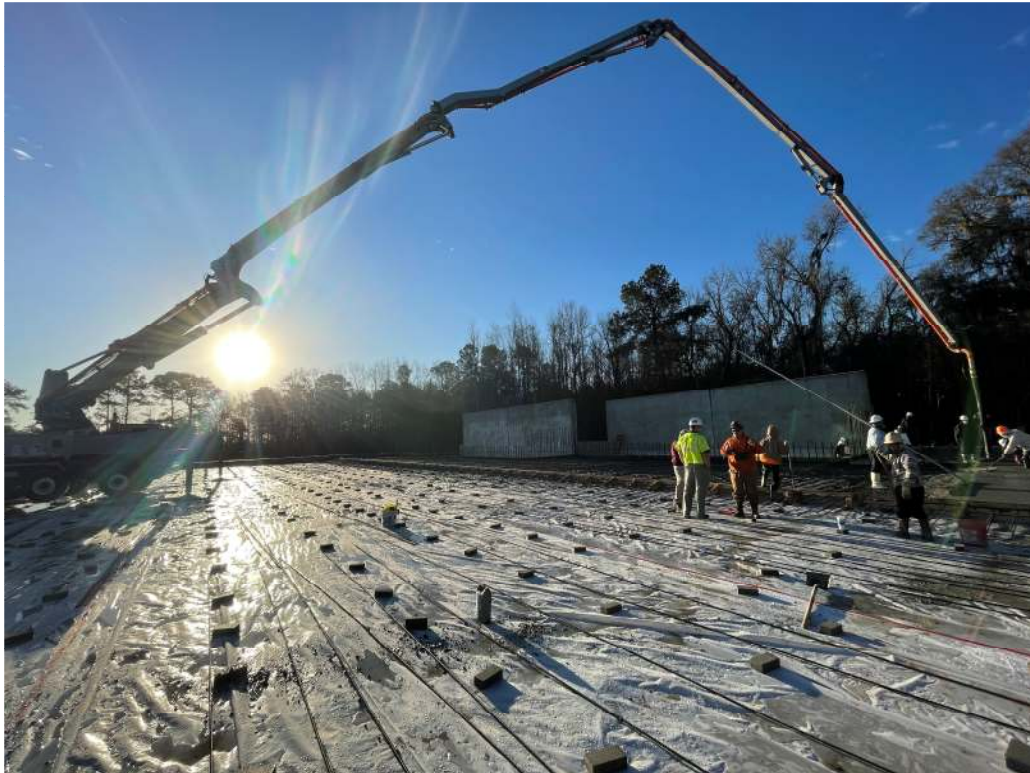
Figure 2. EdenCrete® enhanced concrete slab being installed
