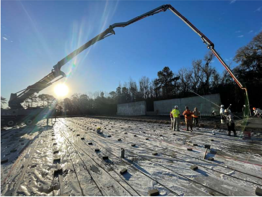
Figure 2. EdenCrete® enhanced concrete slab being installed
