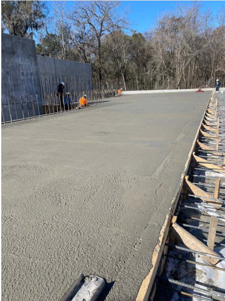
Figure 3. EdenCrete® enhanced concrete slab being installed
