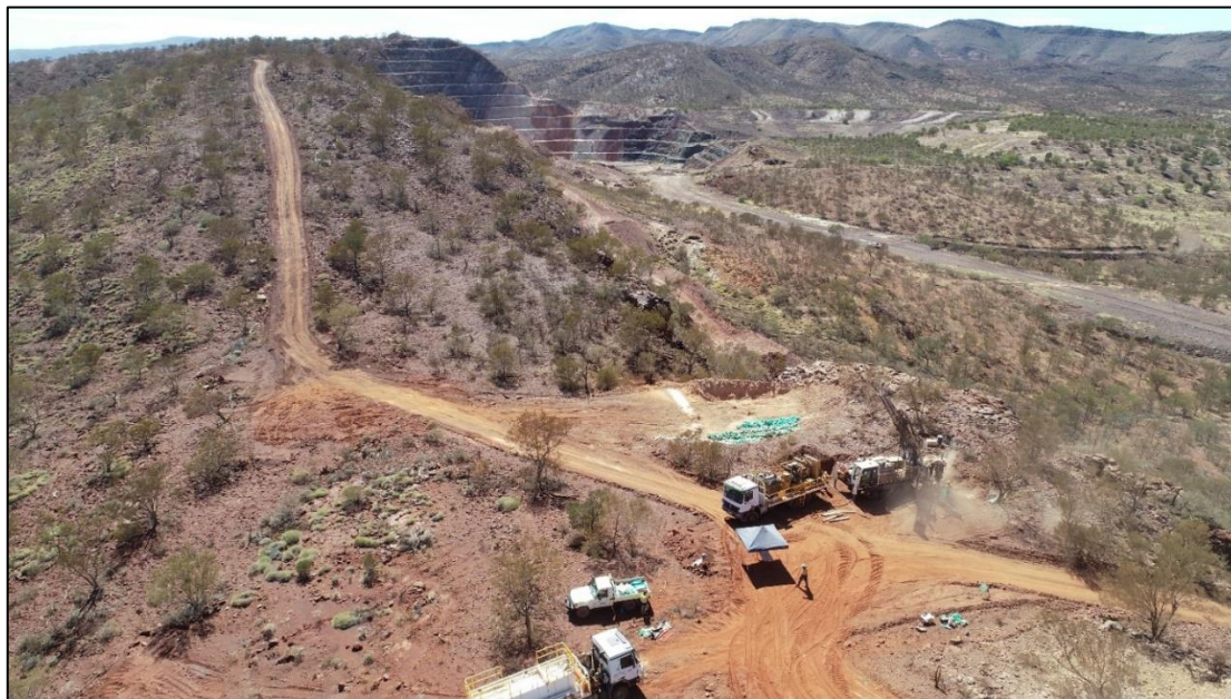
Figure 3: RC drilling at Connie's Find, approximately 400m to the west of the Waugh Pit shown in the background
