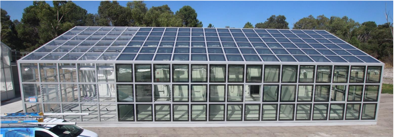
ClearVue's Solar Research Greenhouse at Murdoch University - PV triple glazing installed onto rooms 2,3 and 4 of ClearVue's solar research greenhouse at Murdoch University, Western Australia. Room 1 –a trial 'control' room (far left) showing single pane glazing only.
