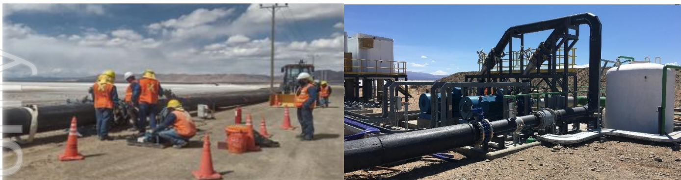
Note: brine gathering network under construction and gathering pond TK1100 pumping station
