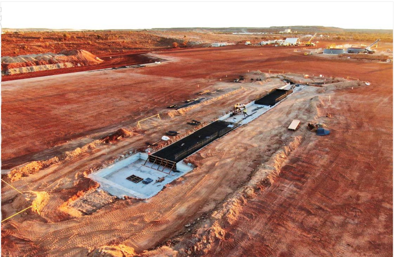
Figure 5: Foundations commenced for stockpile tunnel and reclaim.
