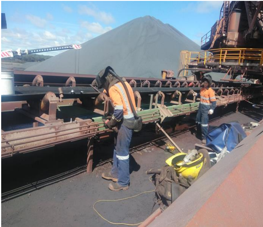
Structural and conveyor repairs at Port Latta
