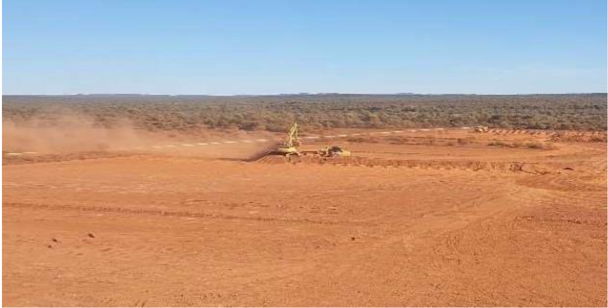
Figure 3. Load and haul of topsoil at site of future processing plant.
