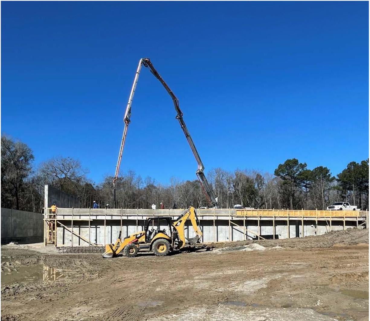
Figure 1. Atlantic Waste Services new waste transfer station
