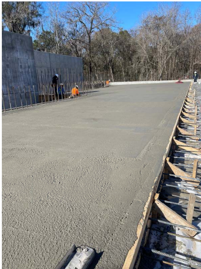
Figure 3. EdenCrete® enhanced concrete slab being installed
