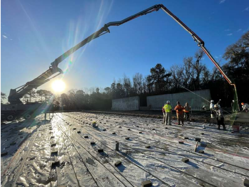
Figure 2. EdenCrete® enhanced concrete slab being installed
