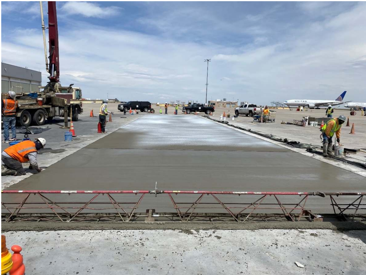
Figure 4 Finishing the 5-panel concrete replacement on United Airlines maintenance hangar apron
