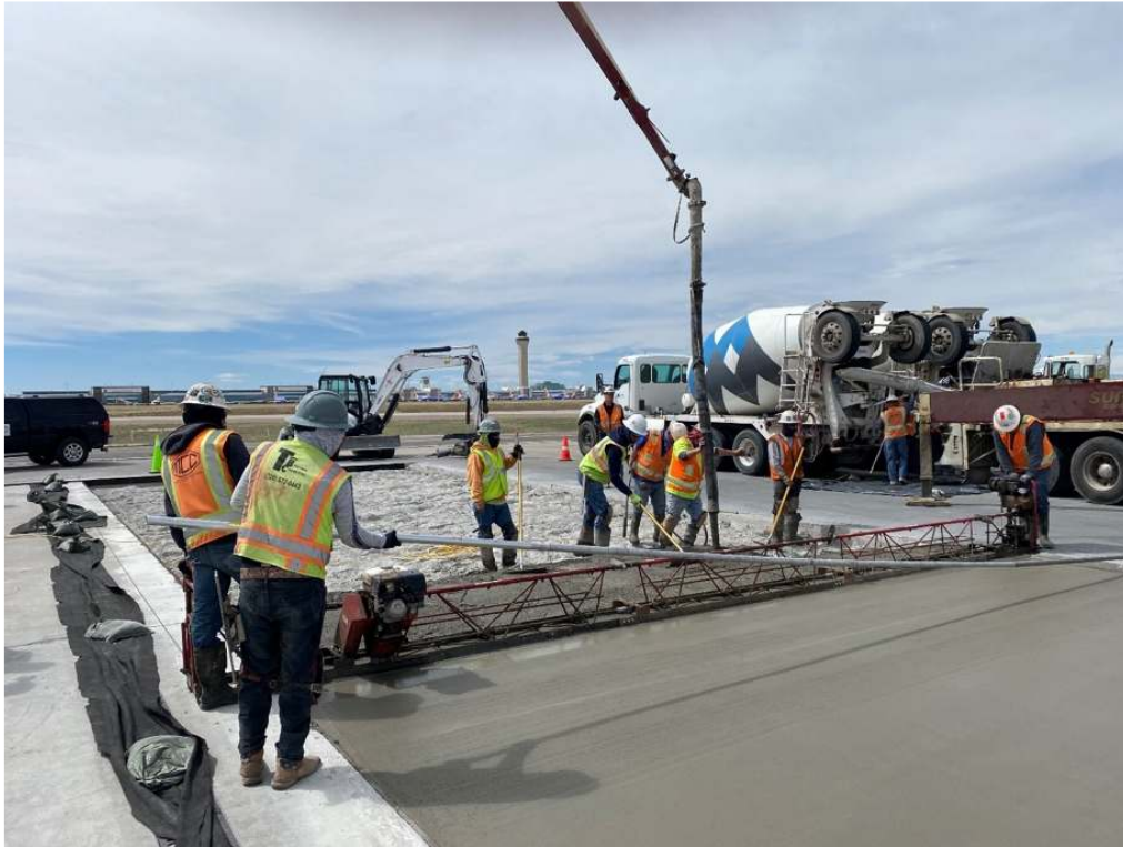
Figure 3 Pouring the replacement concrete panel on United Airlines maintenance hangar apron
