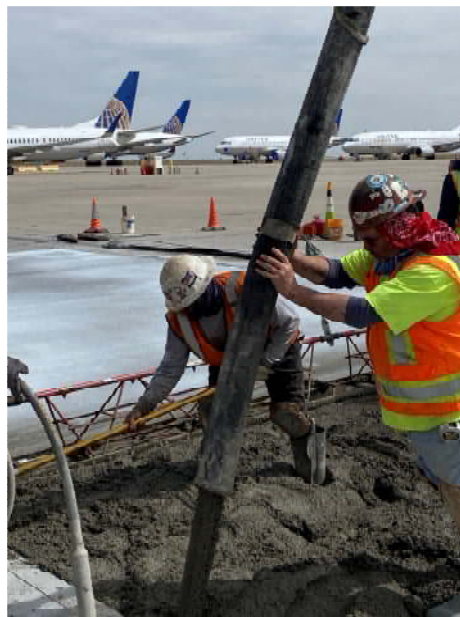
Figure 2 Pouring the replacement concrete panel on United Airlines maintenance hangar apron
