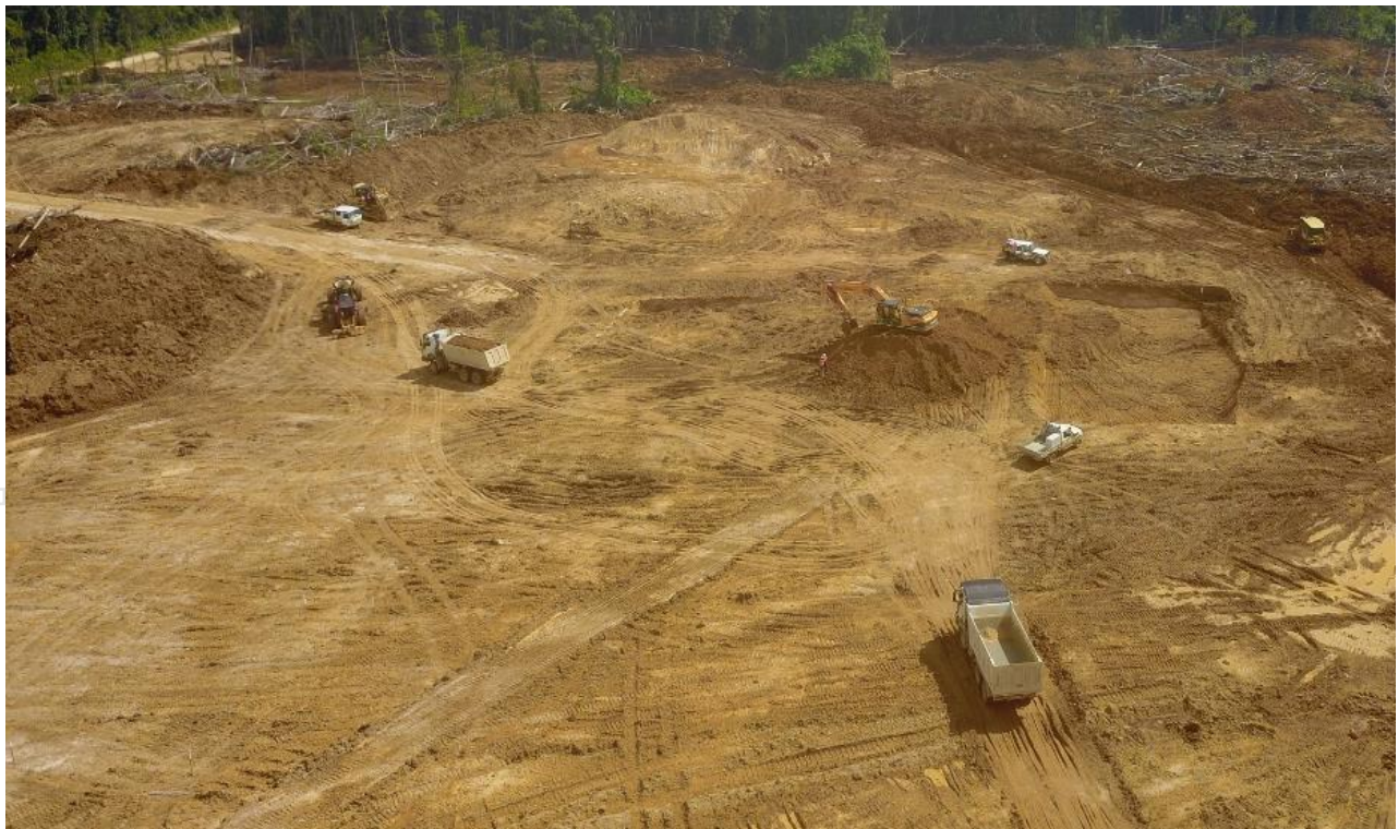
Figure 1: Commencement of processing plant infrastructure: box cut for CIL tanks
