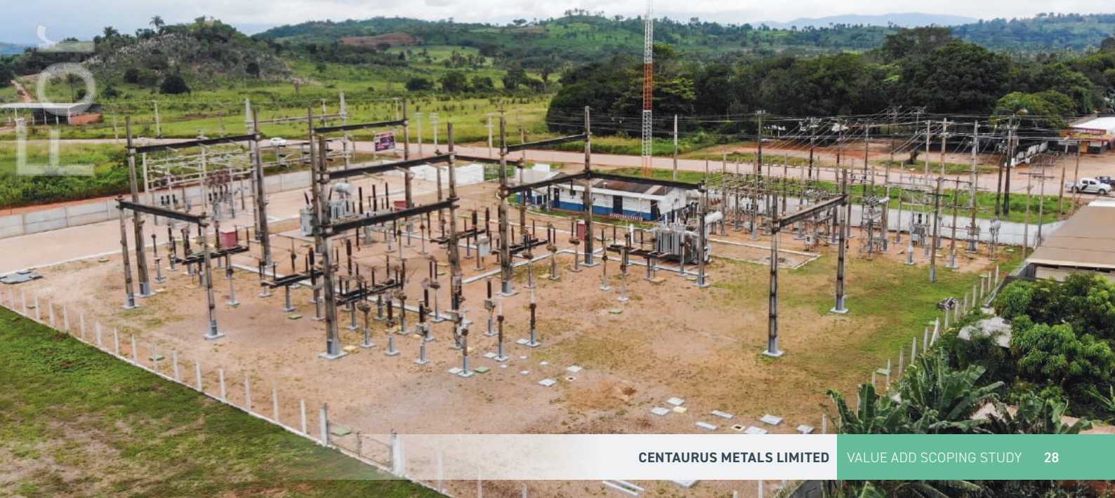
Figure 19 - 138kV National Grid connection at Tucumã
