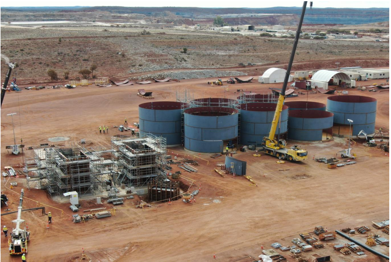
Figure 2: Preparation for the concrete pour of the plinths for the processing plant is underway.
