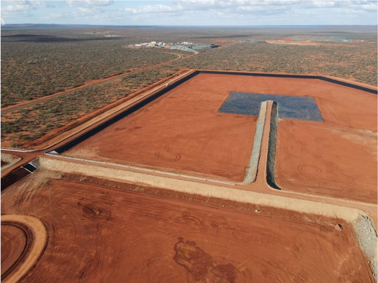
Figure 3: New Deflector TSF
