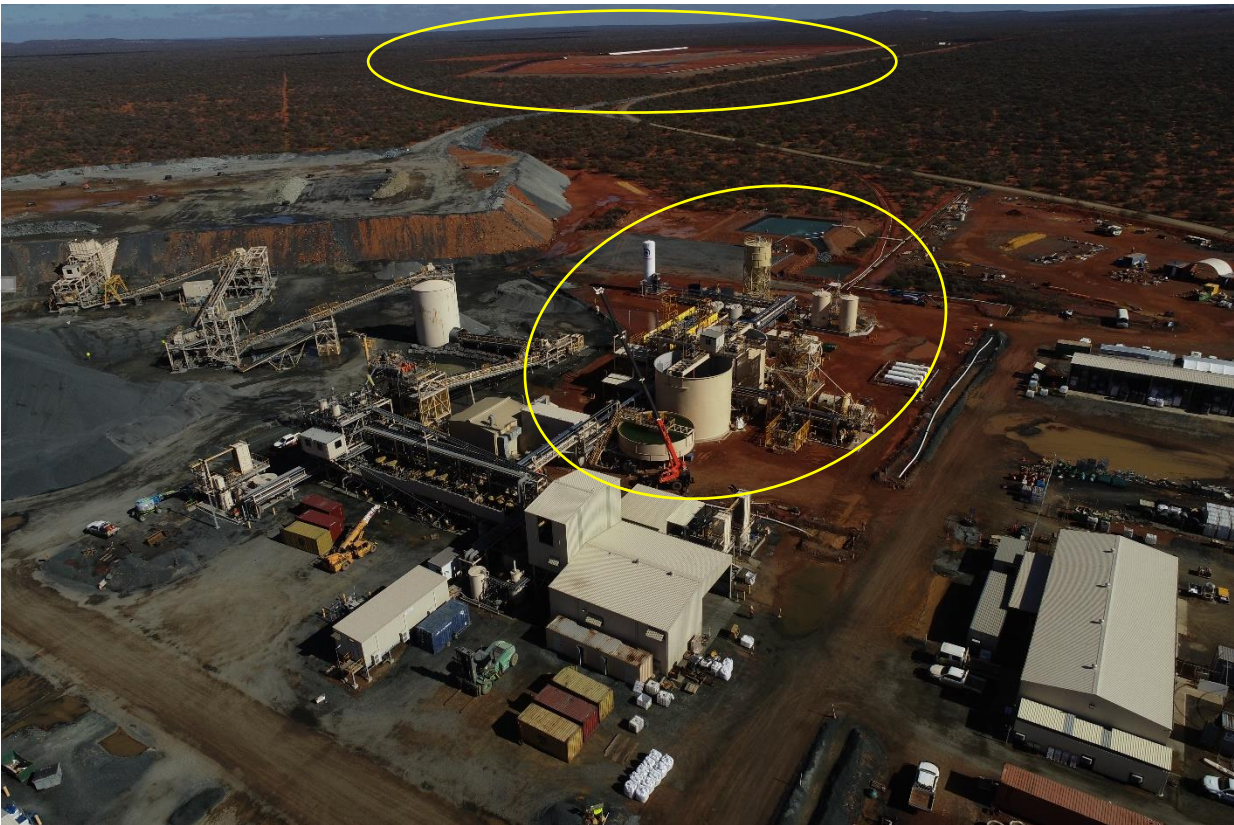
Figure 2: Upgraded Deflector plant and new tailings storage facility (TSF)
