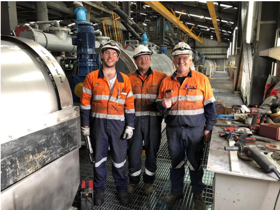
Completion of Rougher Magnetic Separator installation
