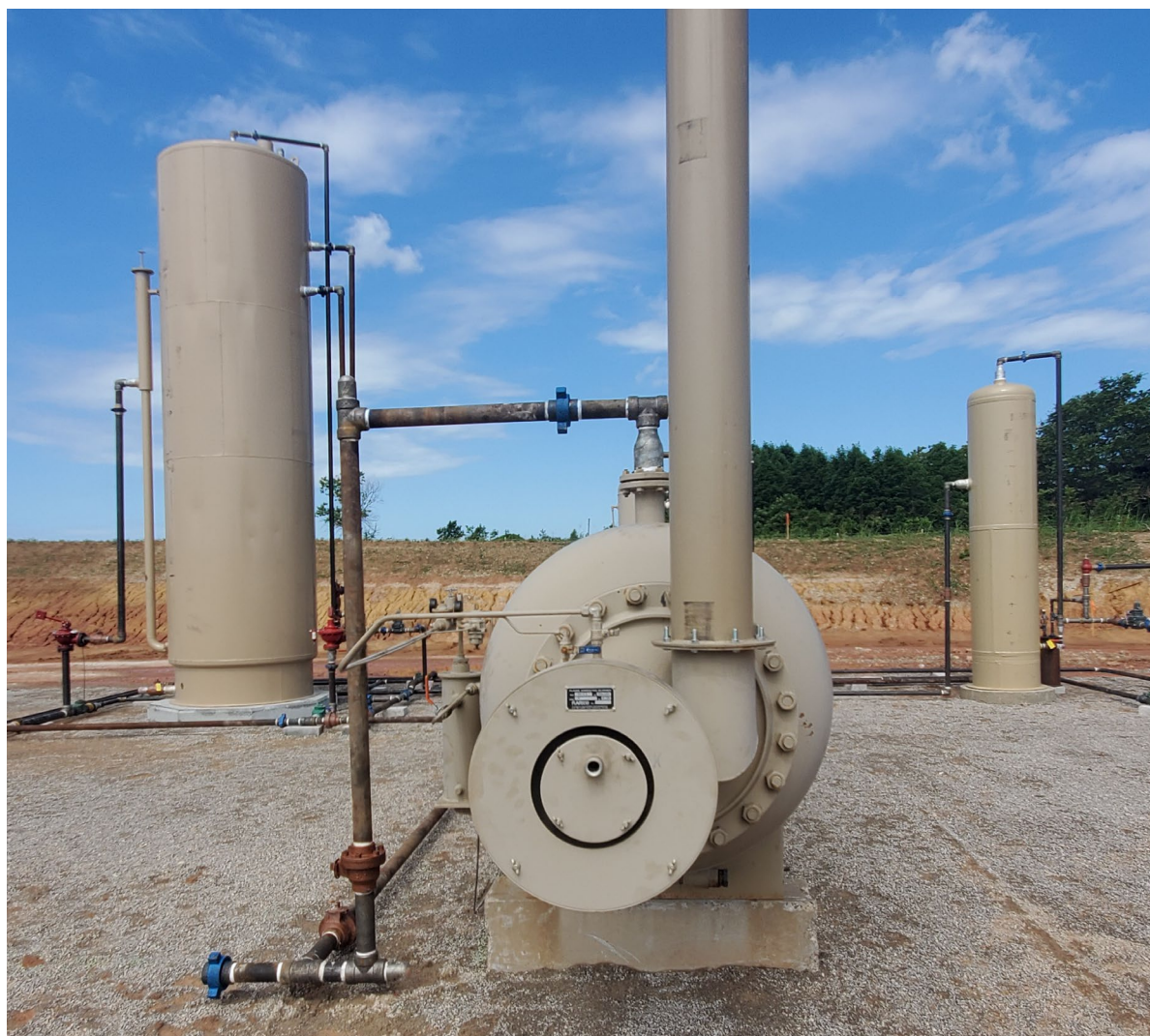
Figure 2: Separators set and plumbed-in on the Jewell Location in Carter County, Oklahoma
