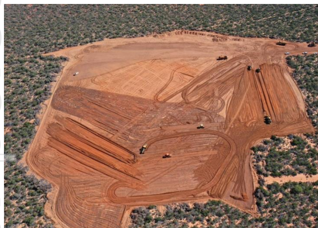
Figure 3 Village Bulk Earthworks Pad
