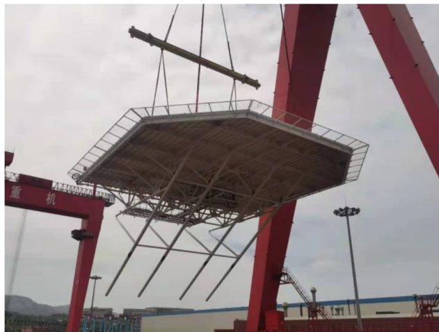
Platform helideck completed and ready for installation
