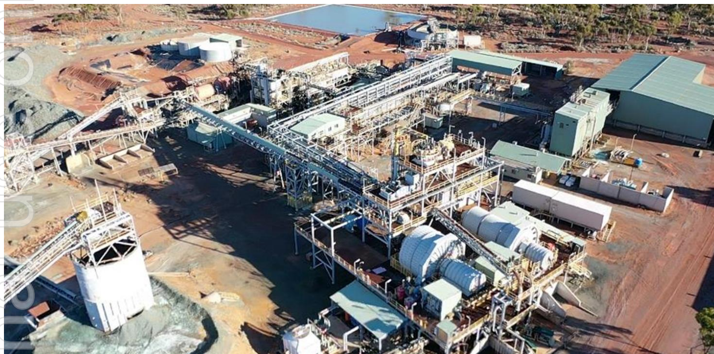
Figure 1 – Black Swan 2Mtpa processing plant with the 150ktpa circuit located between the mills and float circuit
