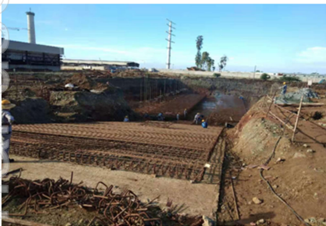
Foundations for Dry Ore shed
