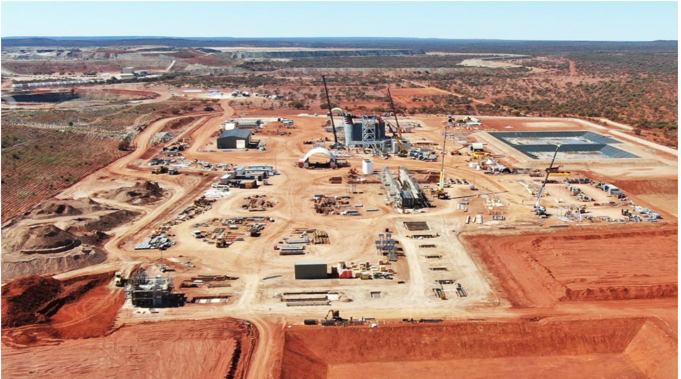
Figure 2: Construction progress at 7 August 2021 – crusher in the foreground, stockpile reclaim tunnel in the centre, mill and CIL tanks at the rear of the photo.
