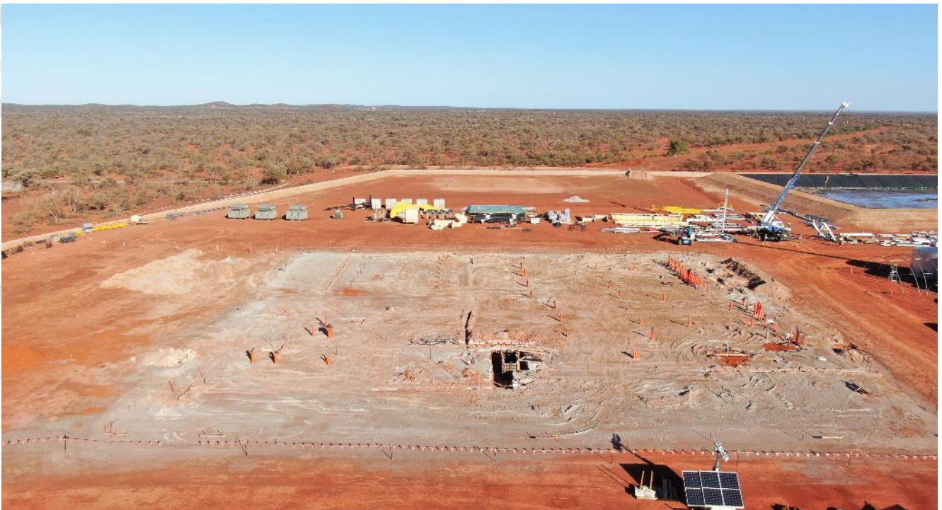
Figure 3: Power station site at 3 August 2021 – trenching, conduit installation, and switchroom/generator hall footings have commenced.
