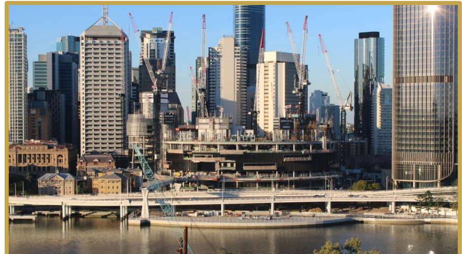
VIEW FROM SOUTH BANK – AUGUST 2021
