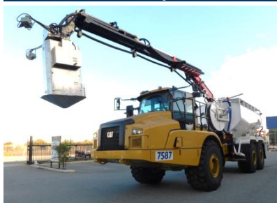
Robotic explosive placement
