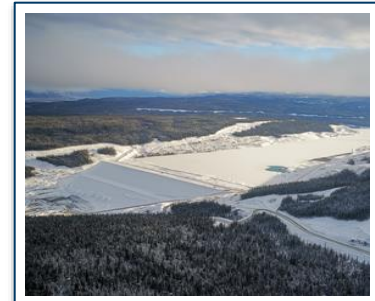
Transition to cyclone sand construction for Tailings Impoundment Area dams underway
