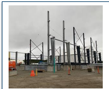
Continue to upgrade facilities, with the construction of life of mine maintenance and combined office buildings
