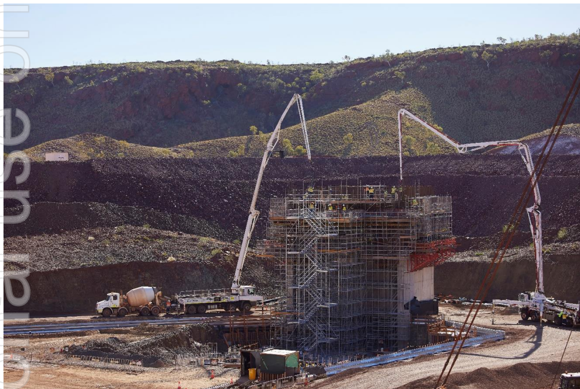
Construction of primary crusher
