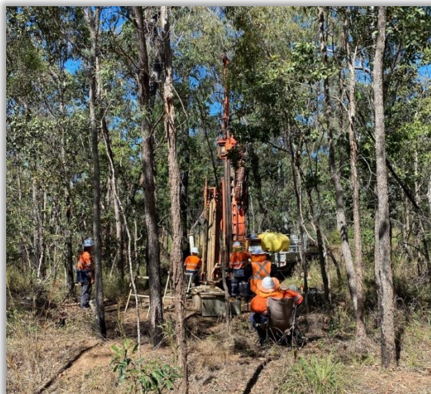
Geotechnical drilling – HPA First Project Site Gladstone
