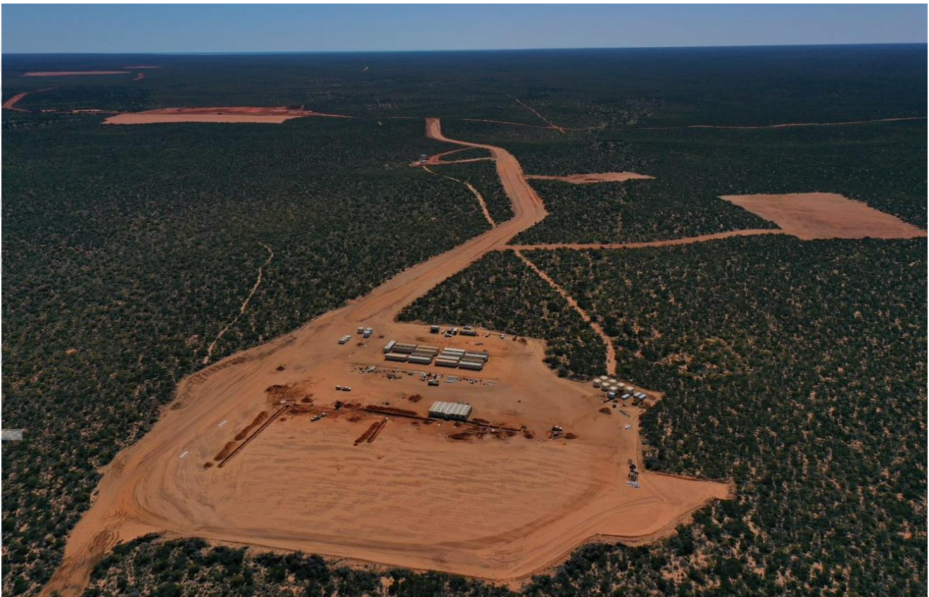
Figure 12 Earthworks Clearing Completed for all Infrastructure Areas including village, MSP, WCP and Bore Fields
