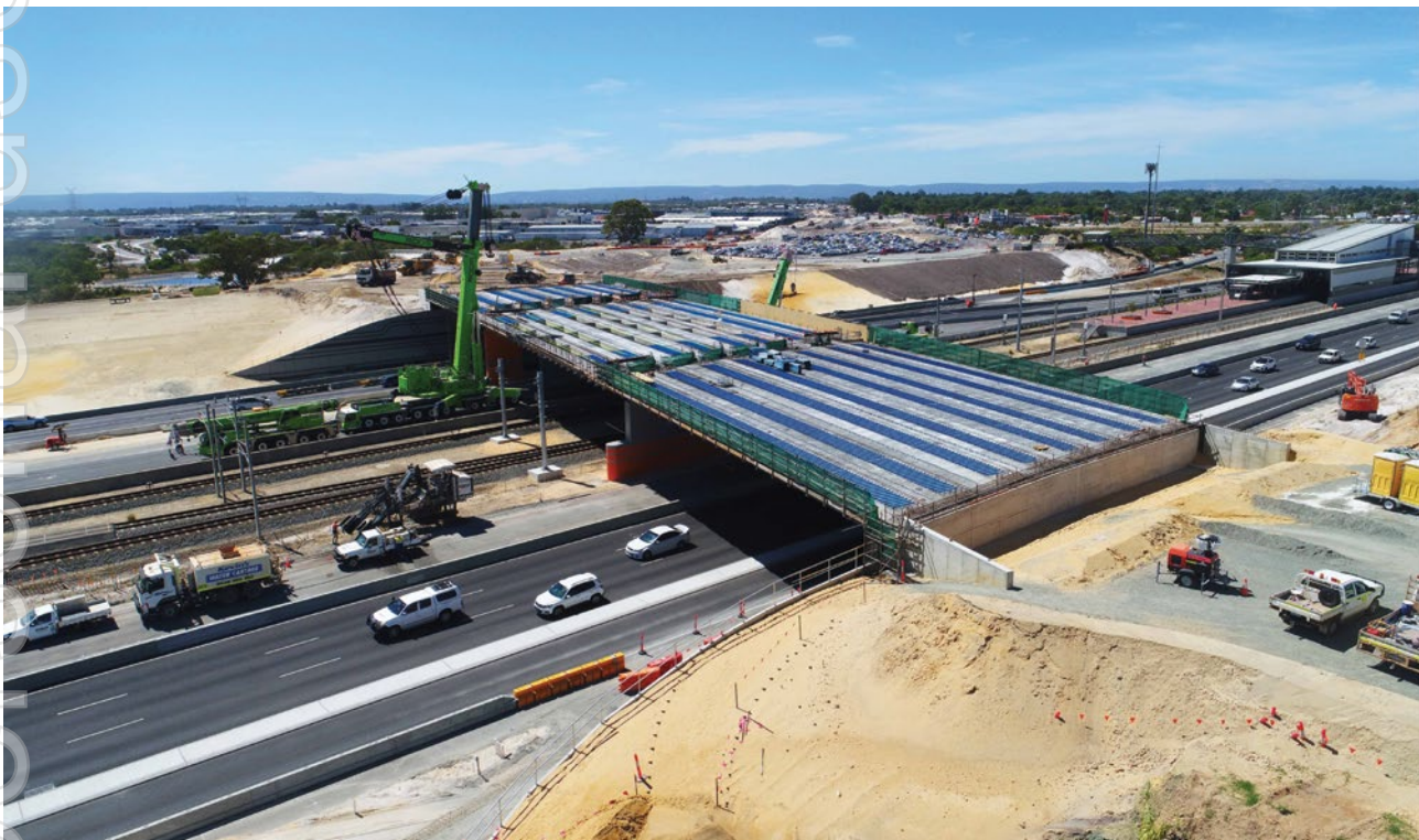
24 bridge beams installed over Kwinana Freeway, between Beeliar Drive and Berrigan Drive (Source: Main Roads Western Australia)
