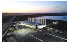
Ravenhall development, Melbourne
