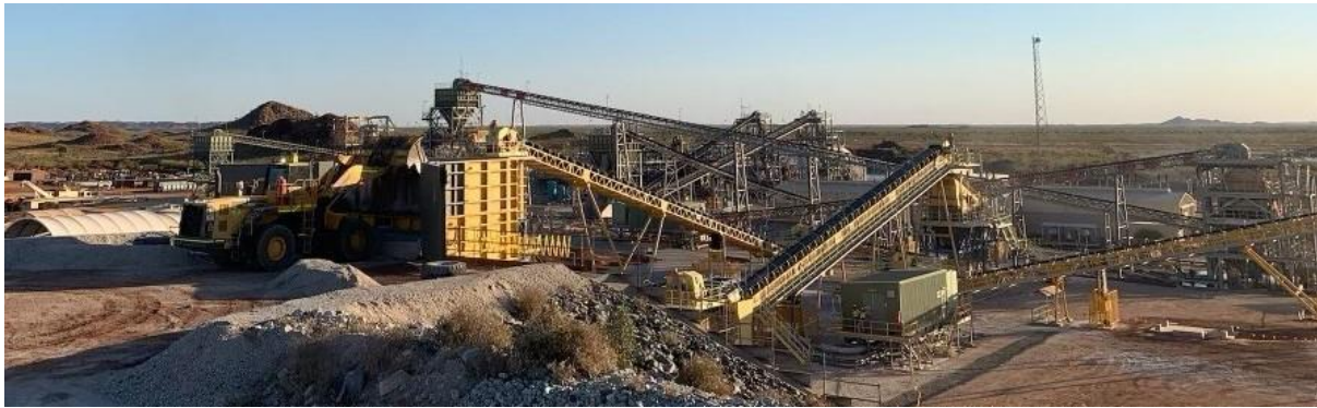
ORE FEED TO THE NGUNGAJU CRUSHER IN SUPPORT OF PLANT COMMISSIONING
