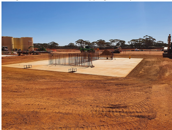
Kiln pad and pier under construction to enable delivery of the kiln shell
