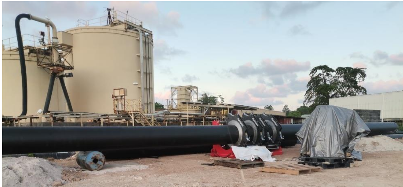
DSTP pipeline - welding of first two pipe sections
