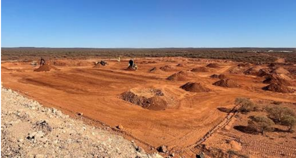
Figure 1. Process plant area bulk earthworks in progress (photograph date 7 th October 2021).
