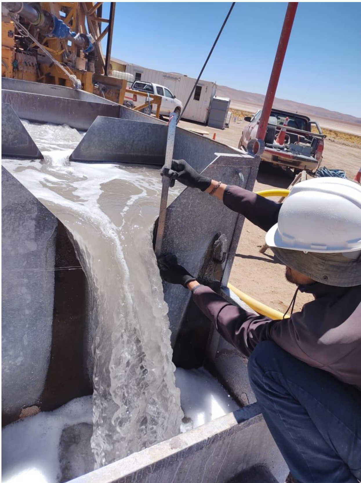
Figure 4: Pata Pila (PB-01-21) bore being cleaned from the previous adjacent drill hole PP-01-19.
