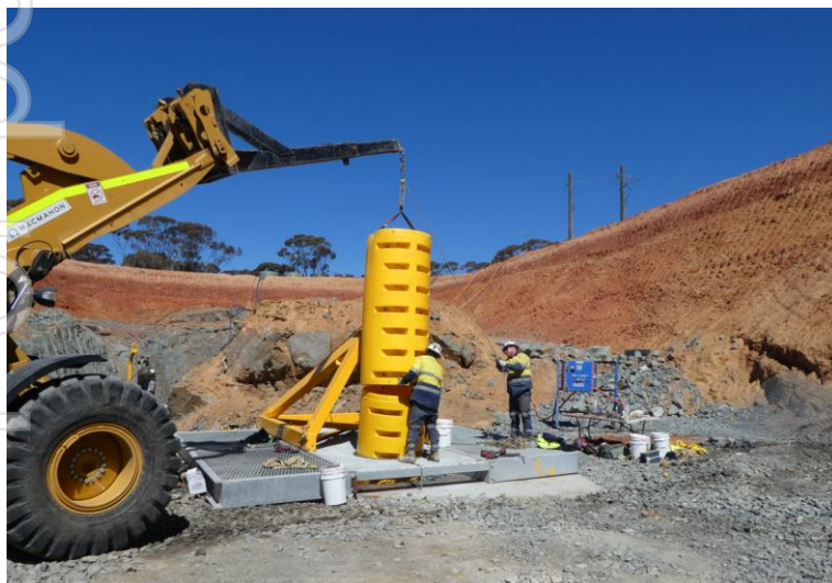
Woodall Decline (L to R) – Escape ladderway being lowered in the box-cut and secondary fan installation for Woodall and Ventilation declines.
