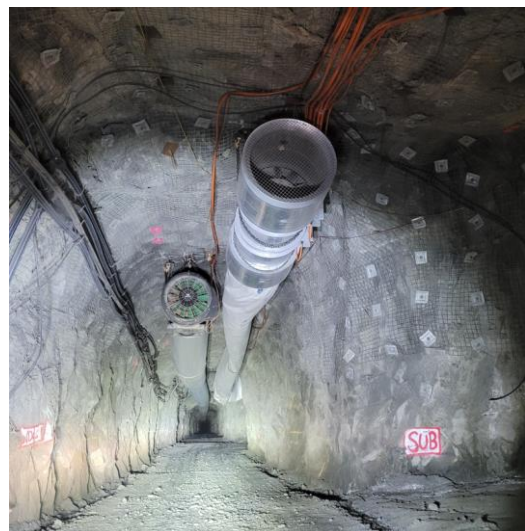
Woodall Decline (L to R) – Escape ladderway being lowered in the box-cut and secondary fan installation for Woodall and Ventilation declines.
