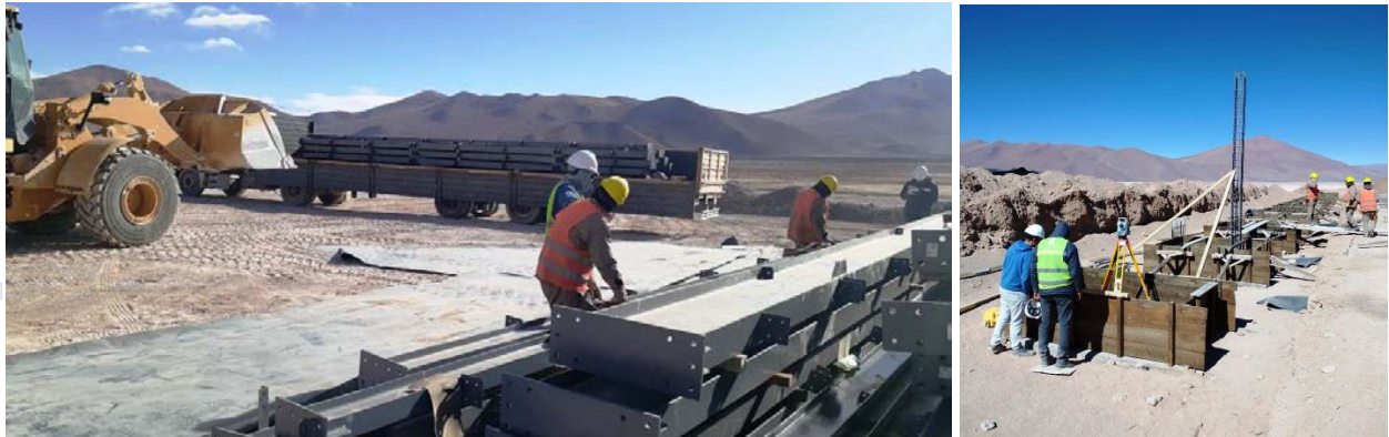
Figures 4-5. Rincon Lithium Project – 2,000tpa Operation Site Works in Progress
