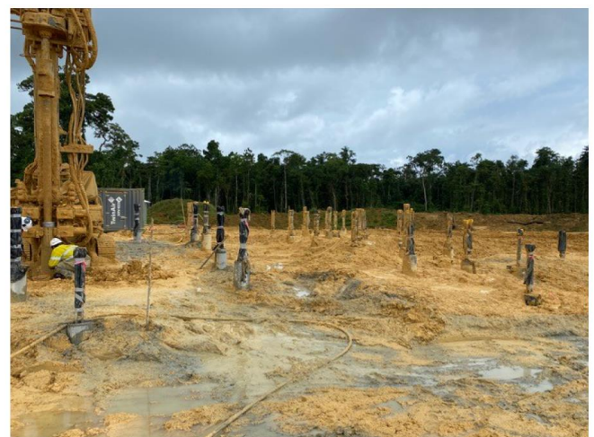
SAG / Ball Mill Micropiling Foundations
