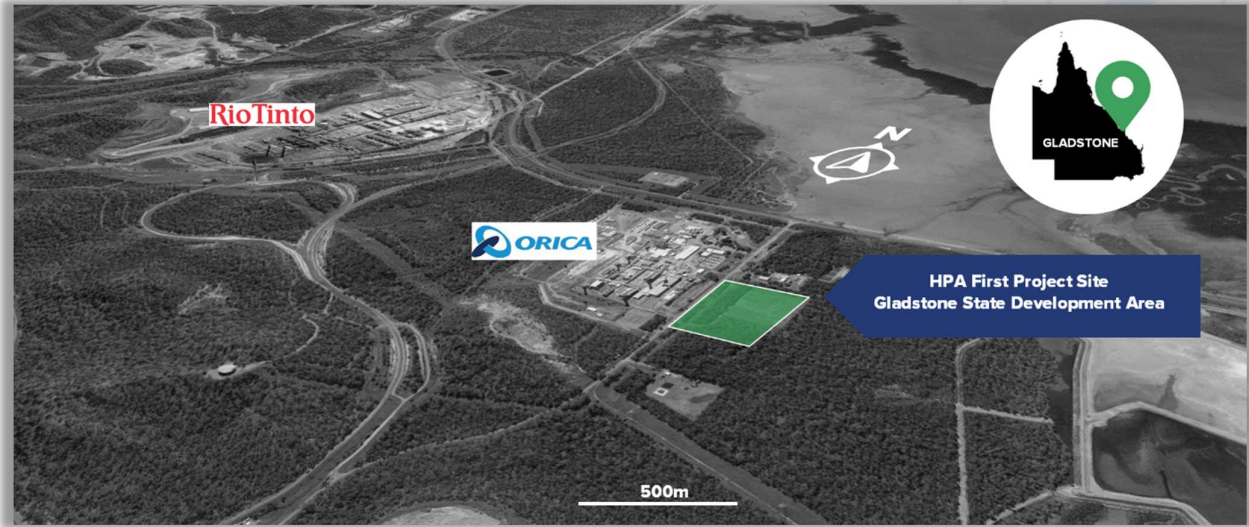
HPA Project Site, Gladstone Queensland
