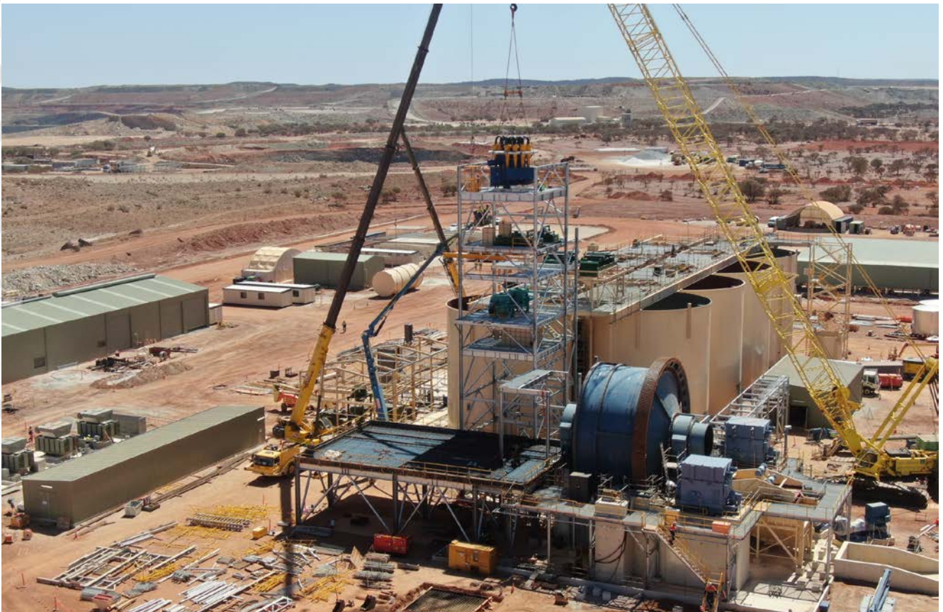
Figure 3: Cyclone being lifted into place at the top of the process plant tower on 2 November 2021.
