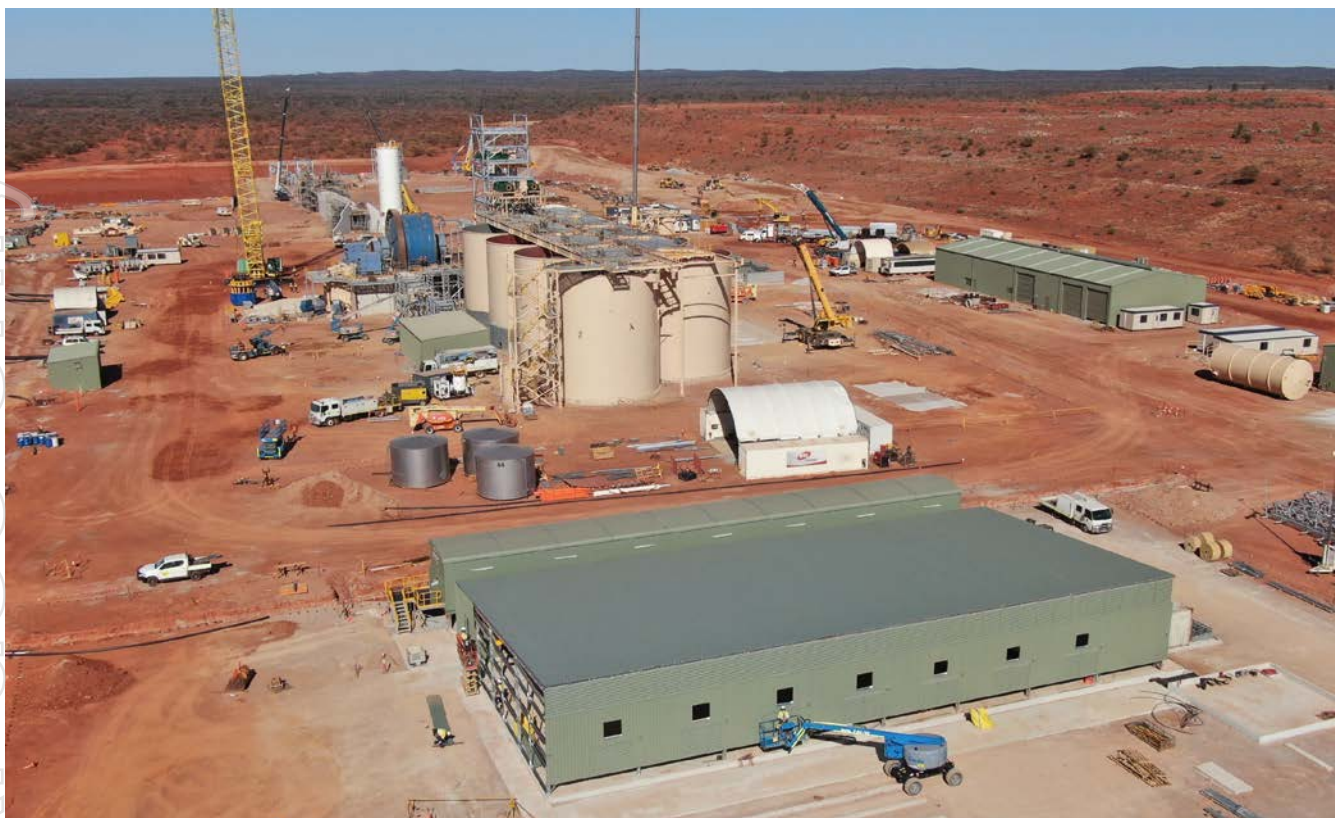
Figure 4: The power station switchroom is installed with engine hall erection nearing completion.
