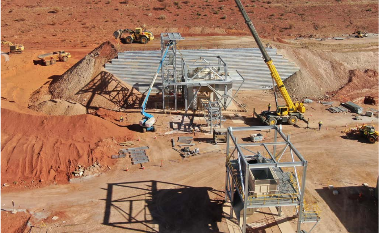
Figure 2: Gyratory crusher base installed, the main frame assembled, and structure being erected.
