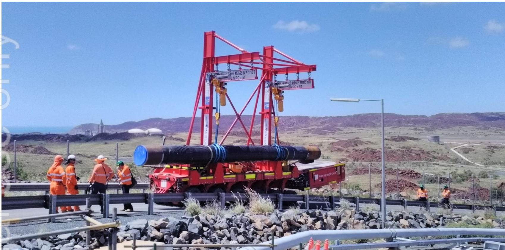
Monadelphous' self-propelled modular transporter Davit frame in operation at the Woodside-operated Pluto LNG Plant, Karratha, WA.
