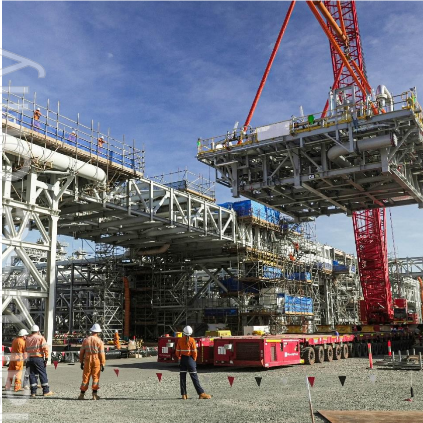
Heat exchanger module being lifted into position at the Woodside-operated Pluto LNG Plant, Karratha, WA.
