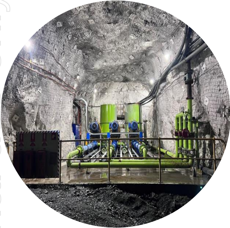
Underground Water Pumping Station
