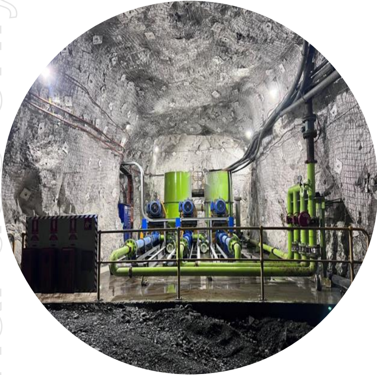
Underground Water Pumping Station
