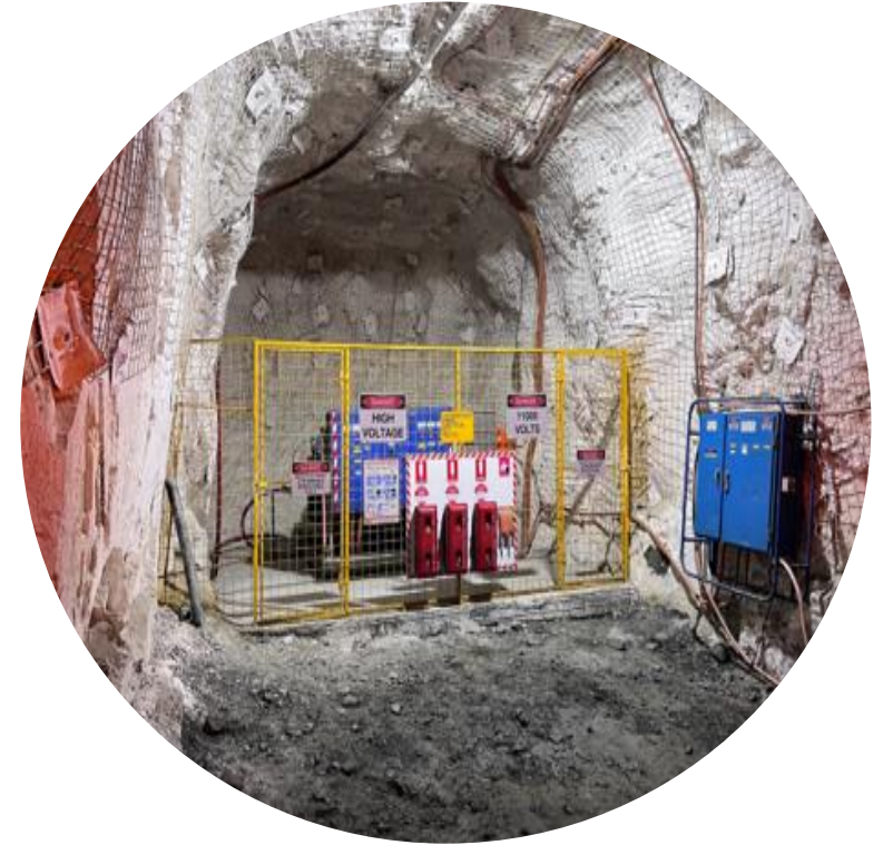
Underground Electrical Substation
