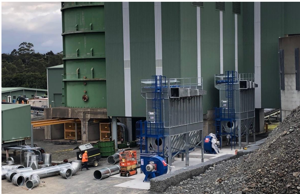
Figure 3. Dust extraction systems adjacent to the Avebury crushing shed
