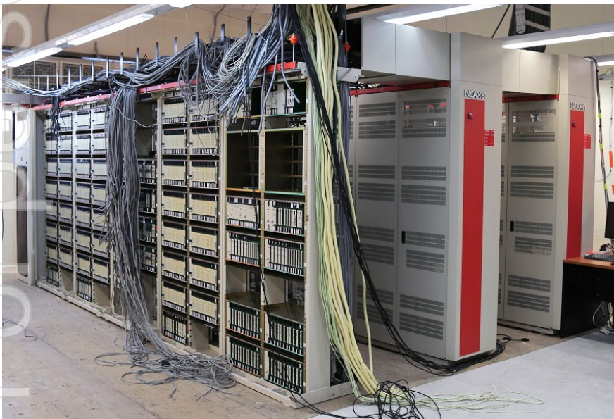
PSTN switches being decommissioned.
