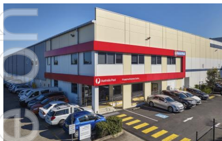
Australia Post, Kingsgrove NSW
