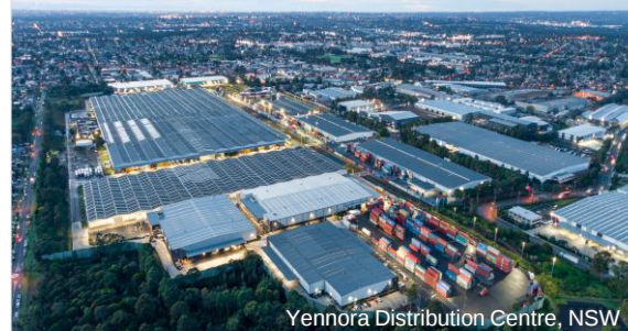
Yennora Distribution Centre, NSW
