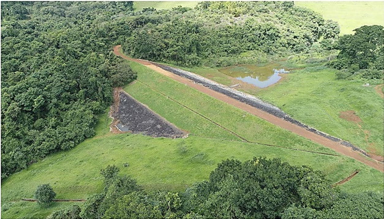
Figure 2 – photo of Dam D. Source: https://cbmm.com/en/our-company/our-dams
